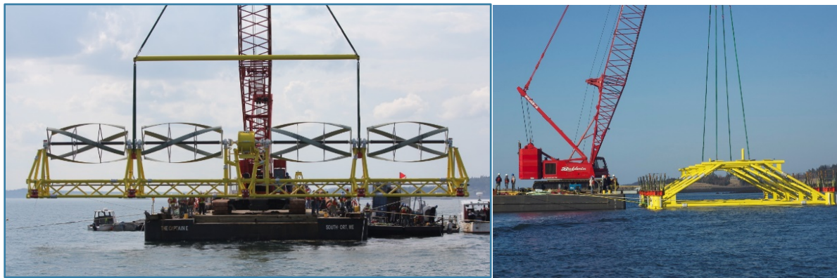
Figure 1. Baseline TidGen® 1.0 (left), deployed over a several weeks period in 2012 with a piled bottom support frame (right). The device produced nearly 85 kW of on-device power at a rated flow speed of 2.25 m/s and had a normalized LCOE of $13.58 kW/h for the DOE reference site distribution at Admiralty Inlet (186,000 MWh array).
